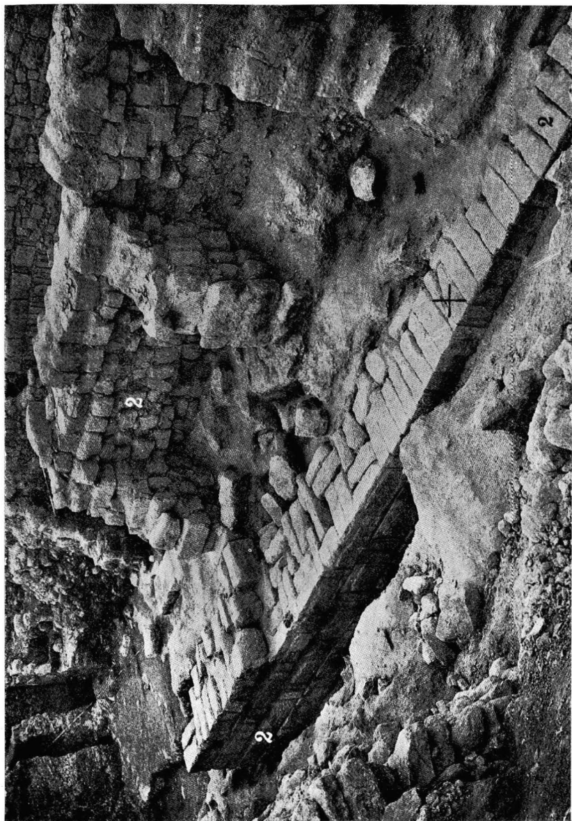
PART OF THE FOUNDATIONS OF AHAB'S PALACE AT SAMARIA.
